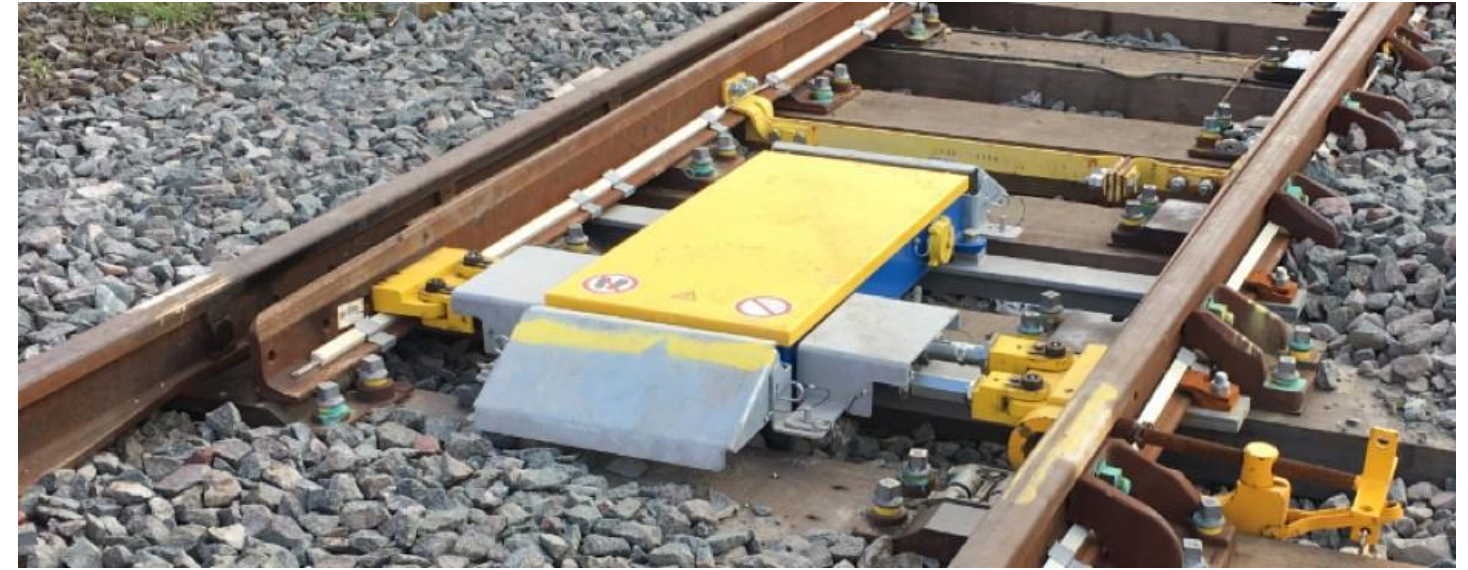
Figure 4 - Point machine installation
