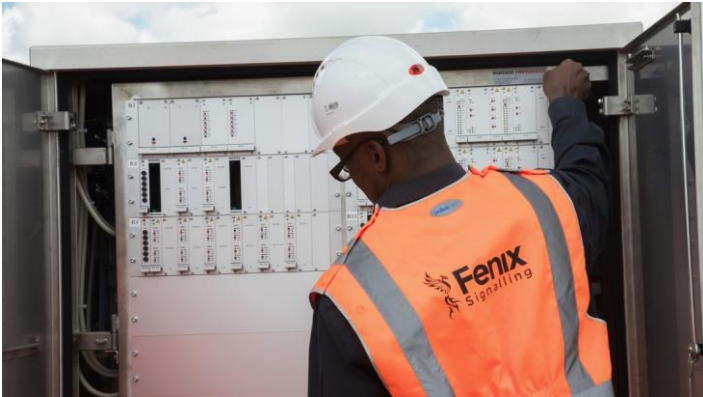
Figure 5 - External location cabinet (frame closed)
