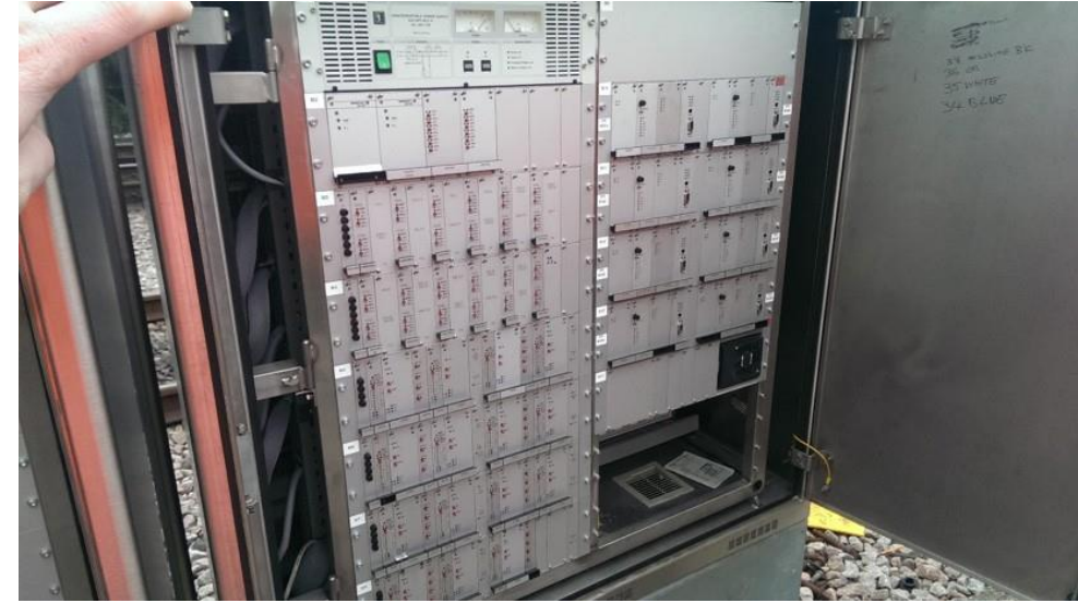
Figure 3 - Interlocking cards (Wembley Depot, SIL 2 only System UK)
