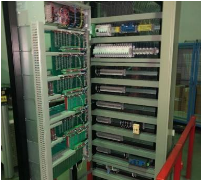
Figure 7 - Wall mounted internal location cabinet (undergoing factory testing)
