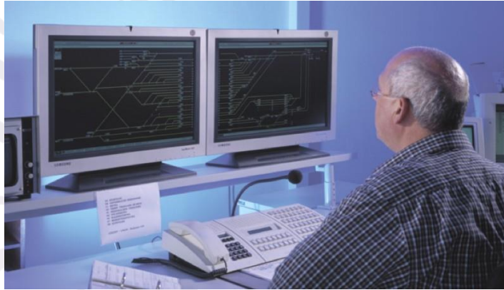
Figure 9 - VDU at Cologne Depot, Germany
